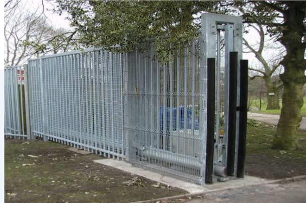
1) Tracked Gates: the sliding-tracked gate runs on a small guide rail set into the surface of the gate opening. The gate includes steel wheels set within the bottom rail of the gate frame which run along the guide rail. The tracked gate requires a perfectly flat and level surface, both across the opening, and for an additional 'run-back' area equivalent to 1.3 times the gate's opening width.
