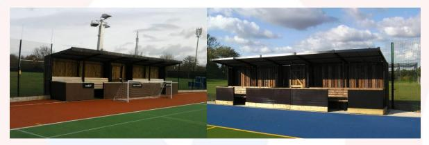
The buildings are constructed from a powder coated steel frame, roofed with colour coated box-profile roofing panels, clad in front with smooth phenolic-faced sports rebound plywood boards (and optional kickboards), and to the rear and sides with rustic overlapping vertical timber boarding. Steelwork and cladding can be coloured to suit the adjacent fencing and/or synthetic carpet.
