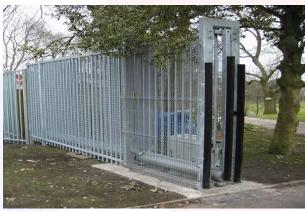
1) Tracked Gates: the sliding-tracked gate runs on a small guide rail set into the surface of the gate opening. The gate includes steel wheels set within the bottom rail of the gate frame which run along the guide rail. The tracked gate requires a perfectly flat and level surface, both across the opening, and for an additional 'run-back' area equivalent to 1.3 times the gate's opening width.
