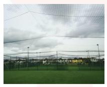
The netting is attached to a series of taught horizontal linewires. Linewires are strained between braced straining posts. Between straining posts the linewires and netting are attached to intermediate posts. Posts are constructed from robust steel sections, and are set into large concrete foundations below ground level. The posts and supporting concrete foundations are fully designed to take account of the particular wind-loading and ground conditions at their intended location.
